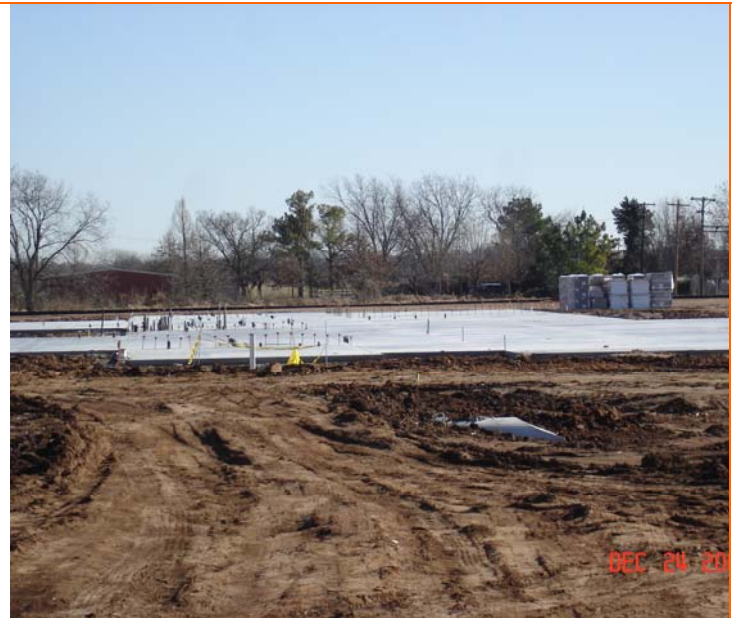
Concrete building slab. This picture was made looking to the east.
